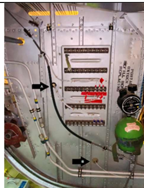
The Bulkhead 4.0 Bomb-Bay Connection Panel was replaced after being removed for refurbishment and to allow the correct location of associated cable runs.
